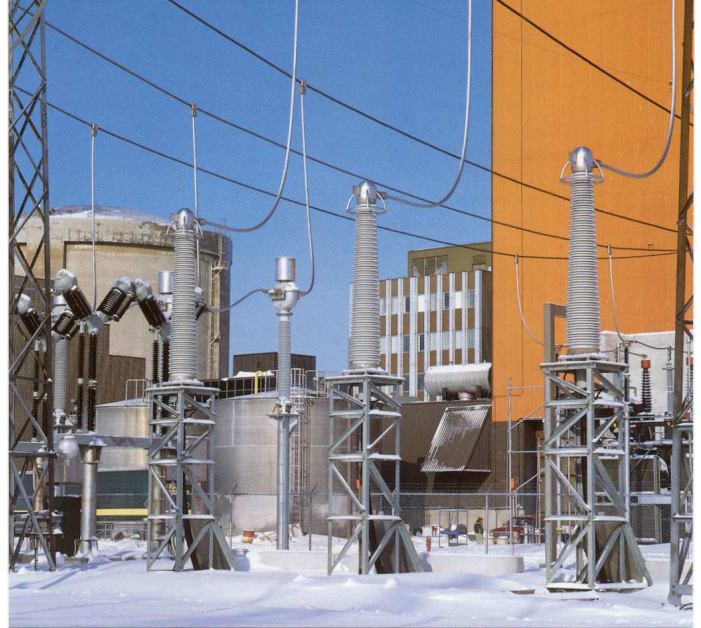
Outdoor terminations in a substation
