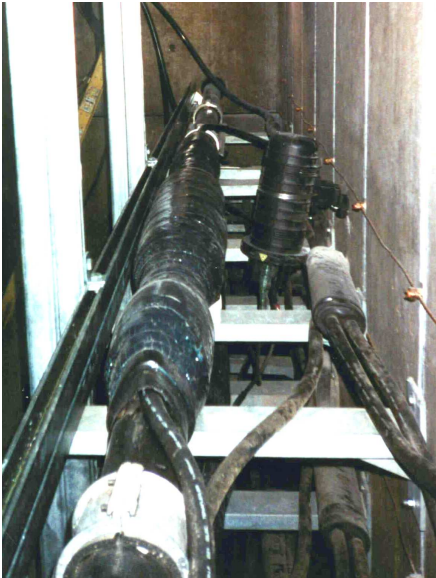
Installation of cable in a vertical shaft
