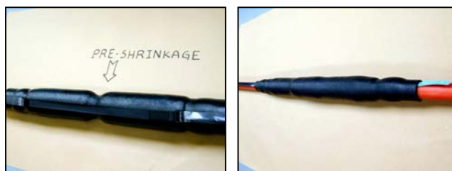
Two step shrinkage of MV joint
